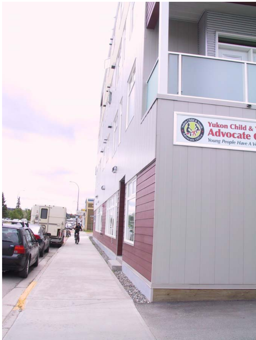
Second Ave Sidewalk next to a 4 Storey Building – the ‘cliff’ effect
