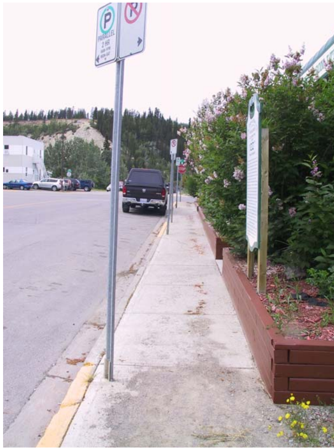
Sidewalk crowded with poles – Hanson and 4th
