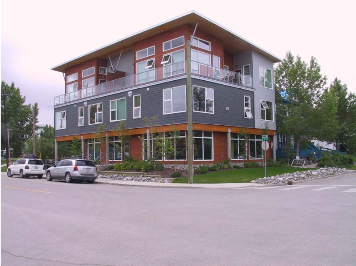
Stepped Building corner of Hawkins and 3 rd . Note also the setback from the sidewalks on both roads.
